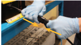
Figure 3: Reconnect AC power to the charger.
