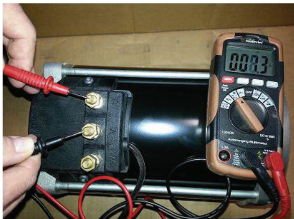
Fig. 21 U and V terminal
