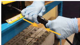
Figure 3: Reconnect AC power to the charger.
